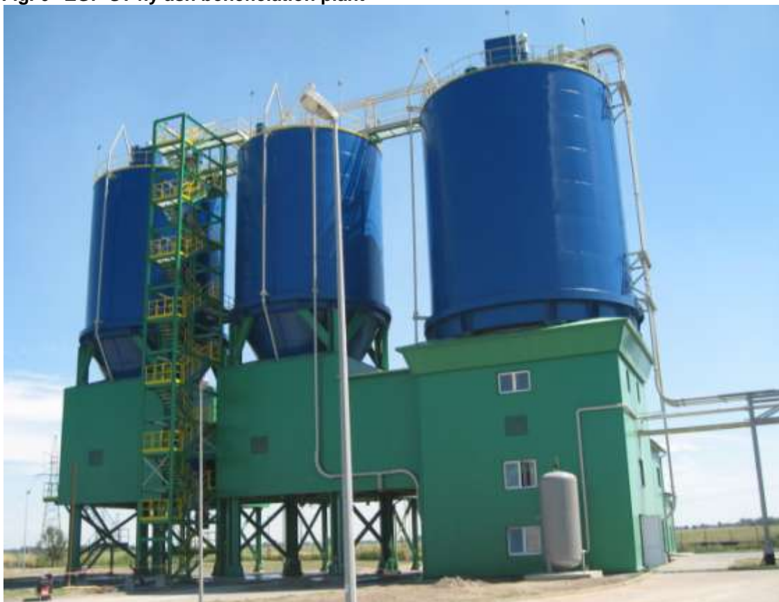
Fig. 6 ZGP ST fly ash beneficiation plant
