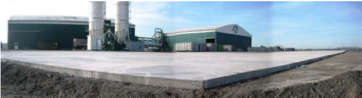
Fig. 3 Base plate with concrete produced with CEM II B-M (W-LL) – MUEG [17]
